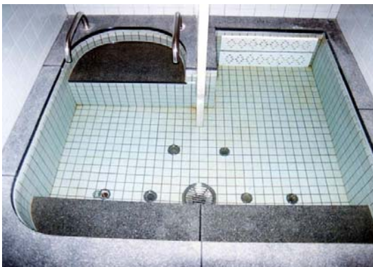
Jacuzzi before installation
