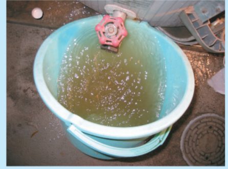
Heated water from the drain outlet: impurities come out toward the end
